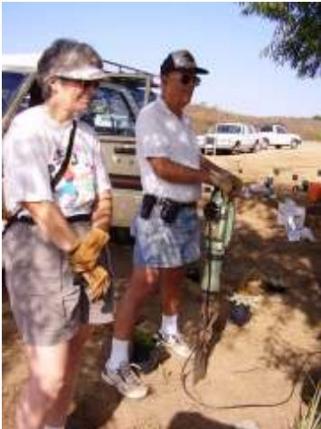
Terry Badger prepares to jackhammer very hard soil
